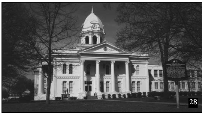
grounds facing Main Street. Historic marker.
